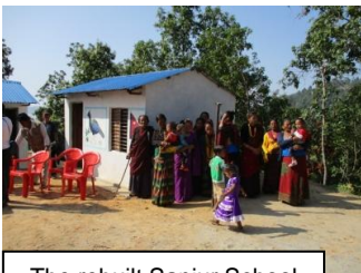
The rebuilt Sanjur School
