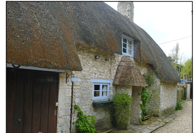
Spinneys, one of Wamsley Lewis houses with low thatch eaves above stone walls
