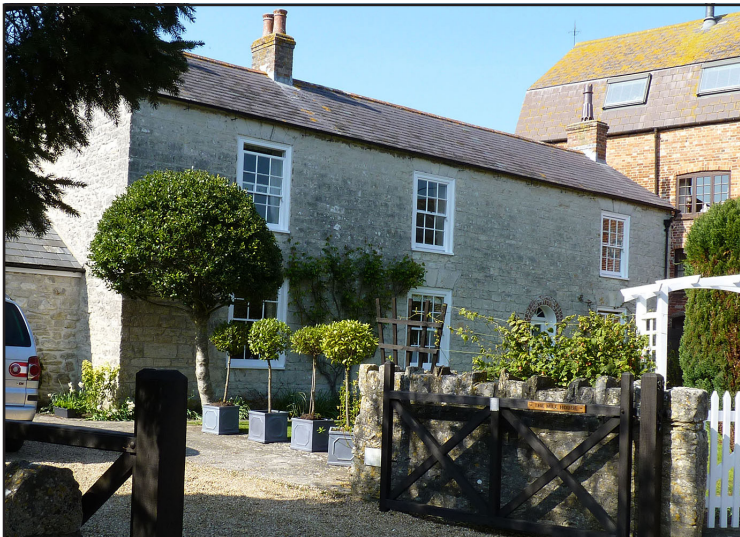
The Mill and Mill House. Stone walls (ashlar at the front and rubble at the back and sides) beneath a slate roof, with good sash windows. The weathered old local brick of the Mill blends in.
