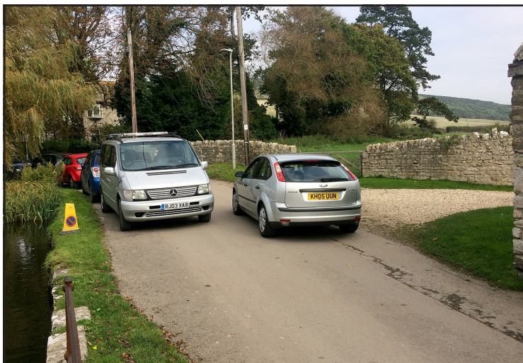
The pond has been damaged by parked cars that also restrict access to the heart of the village.
