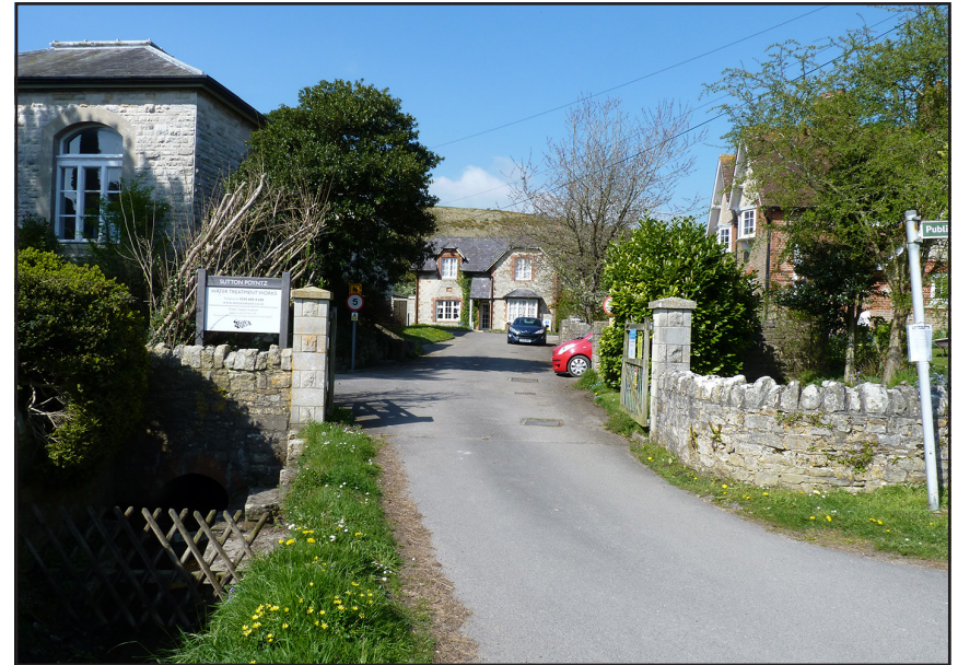
The Waterworks, with 1840's industrial building, 1890's cottages, and the 18th C Upper Mill, represents Sutton Poyntz's industrial heritage.
