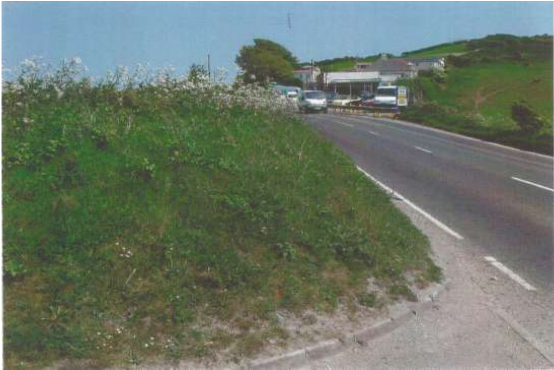
Figure 4 – View up hill to east from access road, showing poor line of visibility
