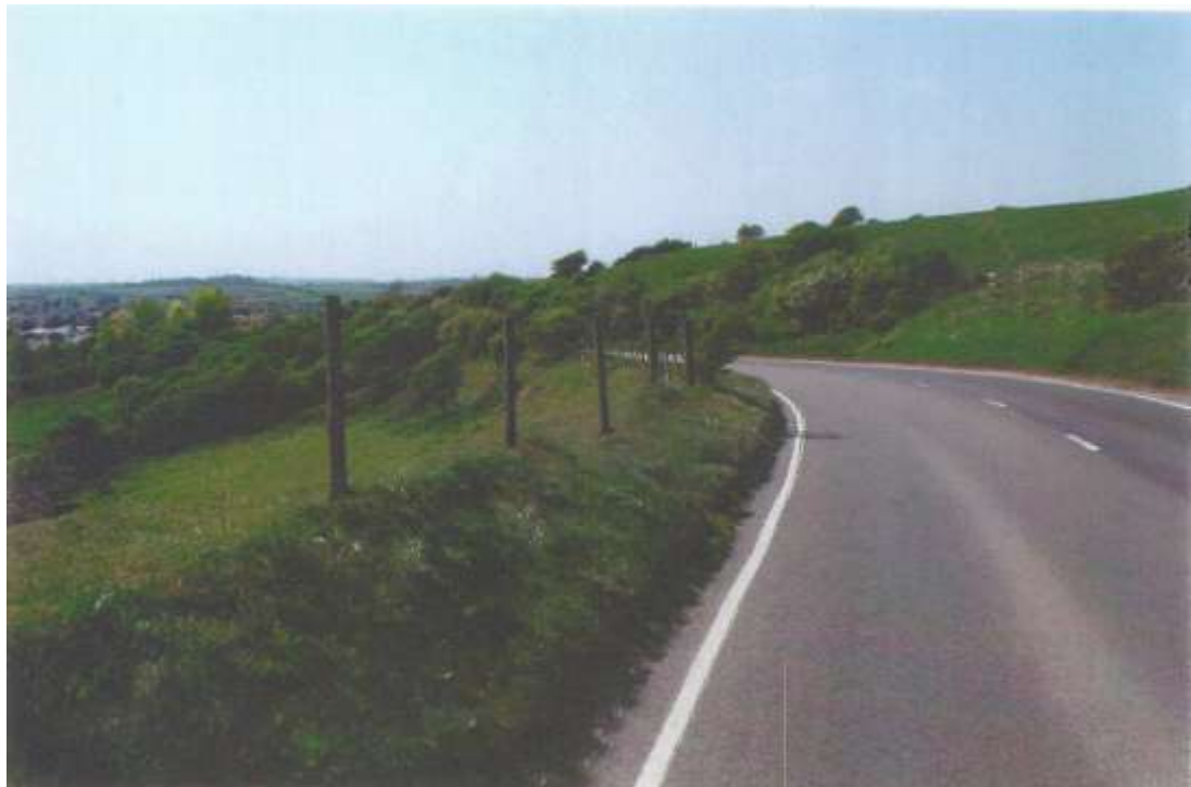
Figure 5 - View along A353, as seen by traffic trying to turn in to access road from the east, showing very restricted view of approaching traffic
