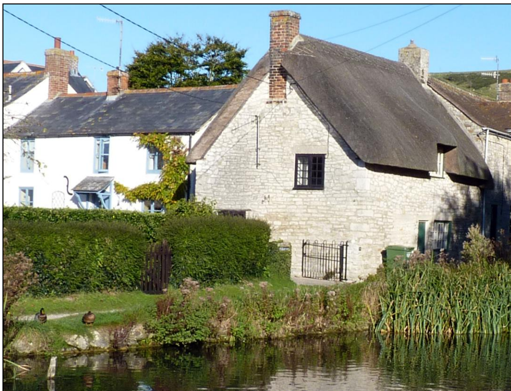
The historic heart of the village, showing rubble stone with thatch and slate roofs
